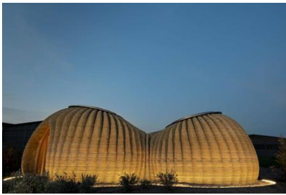
Fig.1 Domed domicile in Bologna, Italy, first 3D-printed construction named “TECLA” (Courtesy WASP)
