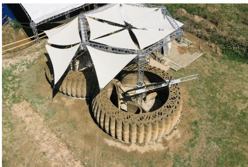
Fig.3 The multi-printer Crane WASP system (Courtesy WASP)
